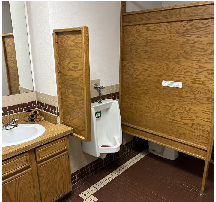
Common Area Restrooms
