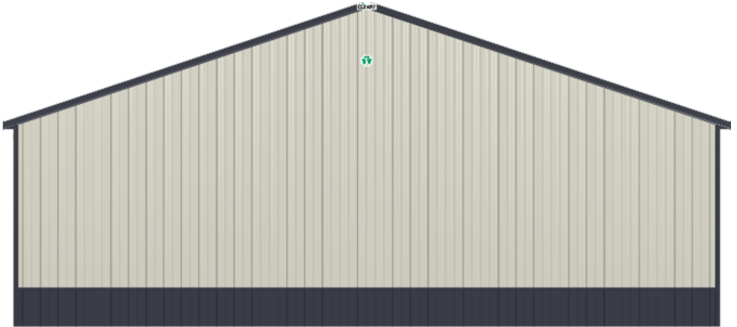
South End Wall 1 on Building 1
